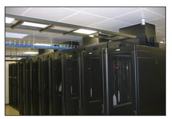
This deployment works with or without divider panels between racks - you can also stack IT load to the top of the rack.
