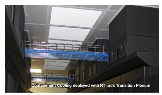
High-density on slab floor, avoidance of cable trays running down or across rows
